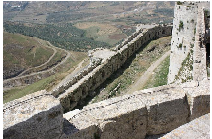
Krak des Chevaliers: standing on the ramparts looking out over the valley
